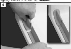
Holding the threshold in place, remove the end cap and mark the end of the rubber threshold with a pencil. Repeat this process on the other end.
