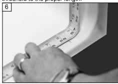
Starting at one end of the rubber threshold, peel back approximately 4-inches of the adhesive backing but do not tear off. Carefully place the threshold on the pencil line at one end and the front alignment line and press firmly in place.
