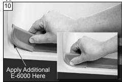
Wipe away any excess uncured adhesive with acetone or a citrus-based solvent.
