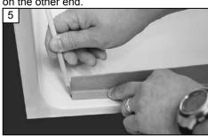
Measure the distance between the two pencil marks on each end and cut the rubber threshold to the proper length.
