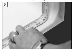
Starting at one end of the rubber threshold, peel back approximately 4-inches of the adhesive backing but do not tear off. Carefully place the threshold on the pencil line at one end and the front alignment line and press firmly in place.
