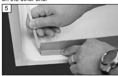
Measure the distance between the two pencil marks on each end and cut the rubber threshold to the proper length.
