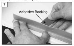
Grasping the adhesive backing previously removed, pull back additional backing, slowly working your way to the opposite end. Make sure the threshold front edge stays on the front edge pencil line, until you have applied the entire length of rubber threshold to the floor. Apply pressure to the entire length of threshold to ensure secure adhesion.
